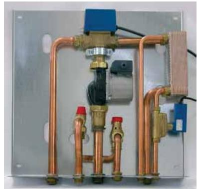
THE INLET AND OUTLET PIPES MUST BE CROSSED FOR THIS TO FUNCTION PROPERLY
